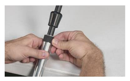
Holding the tee horizontally with one hand on the pipe and one hand on the FlexTop™, slide the rubber tip delicately over the grey ring turning the rubber tip CLOCKWISE as you push it inward over the adhesive.
